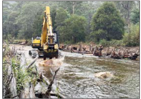
MayFly Rise - Installation of woody habitat
