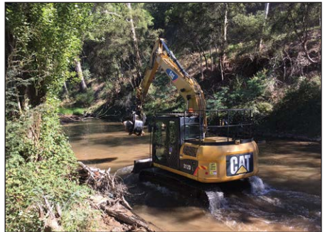
Placement of rocks
