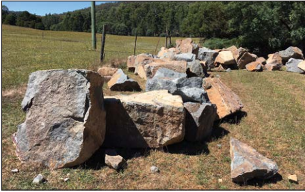
Delivered rocks before placement
