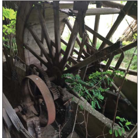
Inside the wheel shed
