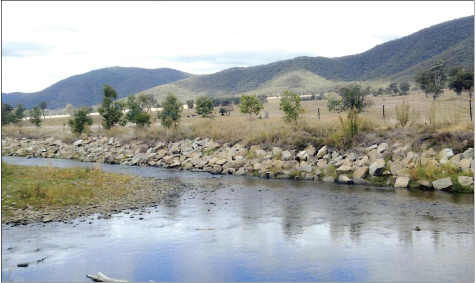
Thowgla Creek, March 2015. The trees have been ripped out and replaced by rocks to stabilize the bank. But no shade for trout and water temperatures in summer rising to lethal levels for trout
