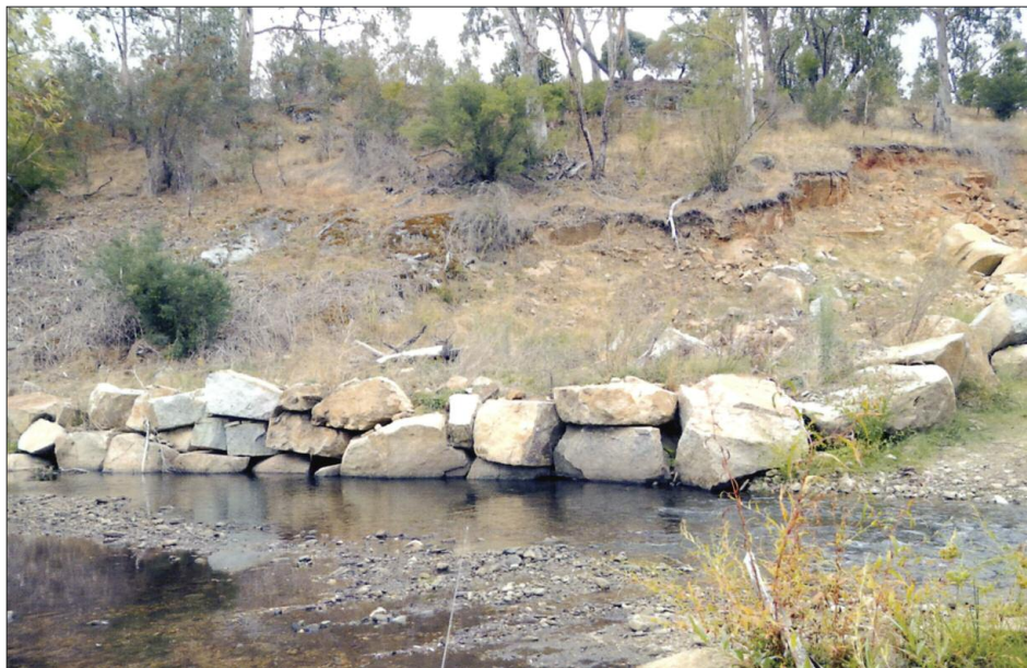
Thowgla Creek, again in March 2015. This pool was once shaded by several willows. Now thanks to 'stream improvement' by the CMA a once attractive and productive trout habitat has been totally destroyed
