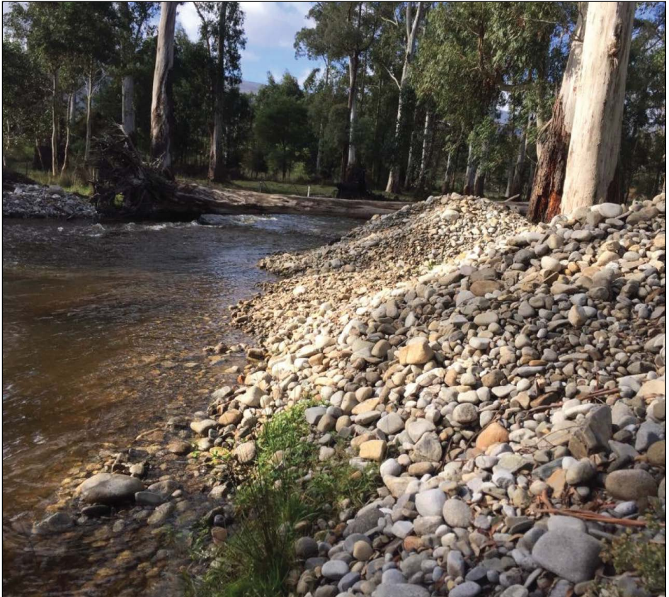
Stevenson illegal waterway works
