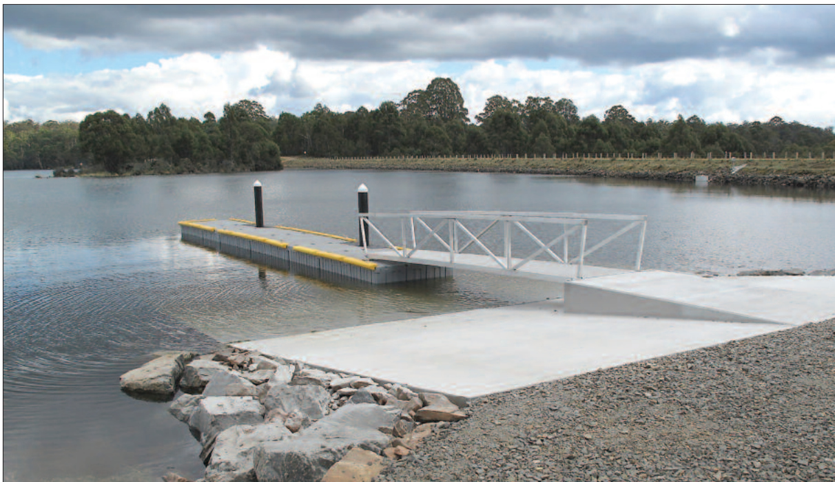
The new boat ramp at Bronte
